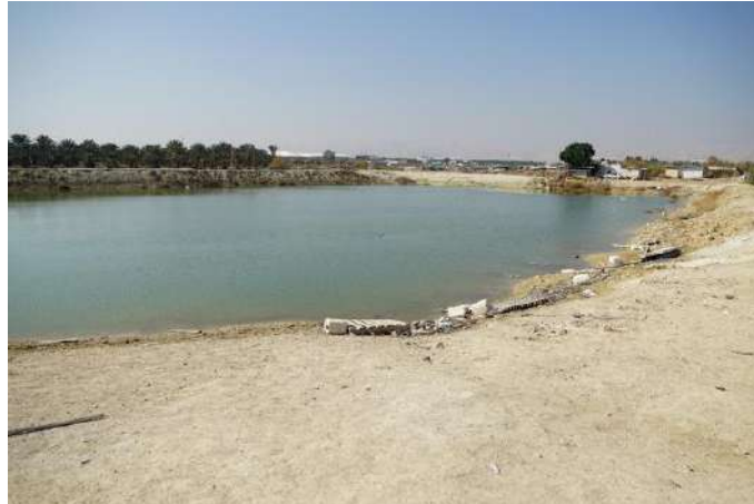
Fig.14 The reservoir used by the MEDISS Project to mix together the waters of different sources
